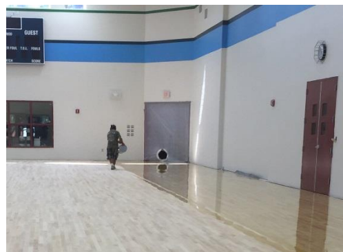
Finishing and Sealing New Gym Flooring
