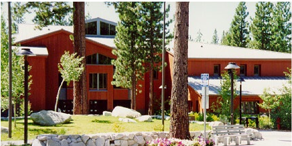
LTCC Main Building
